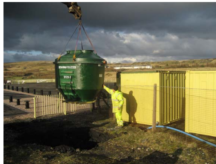
A few days after the storms of 16 January, and with storm clouds still glowering, the Biodigester is buried, safe from threats imposed by the weather
