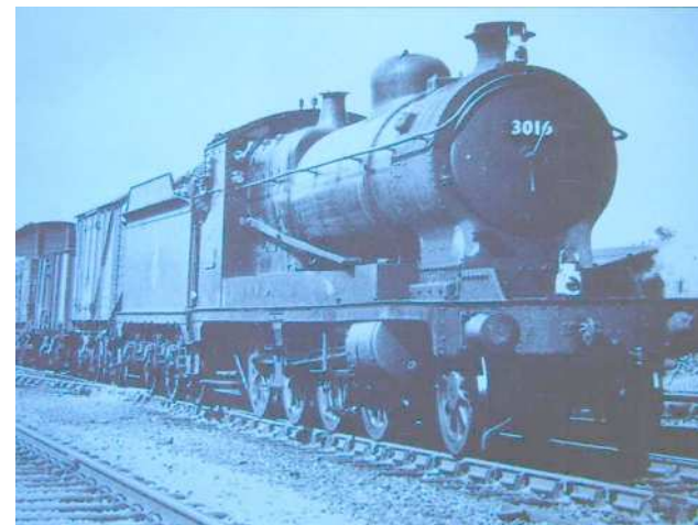
The 1917 RODs were derived from a 1911 Robinson design for the Great Central. Eventually several hundred were in use by the LNER – and classed as O-4s. Several of the 1917 RODs came on to the GWR who couldn't resist fitting GWR safety valve bonnets and other niceties. They were universally disliked by GW men who preferred their own 28xx type. Photo: Bernard Morton
