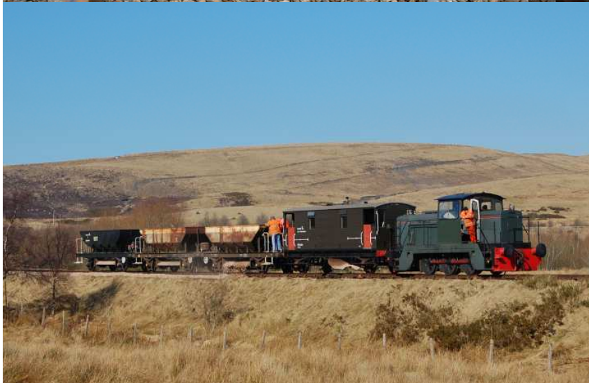
Ballasting by the Whistle Inn, fresh ballast can be seen below the dog fish.
