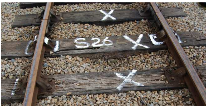
Frost damaged sleepers on the running line. Andy May
