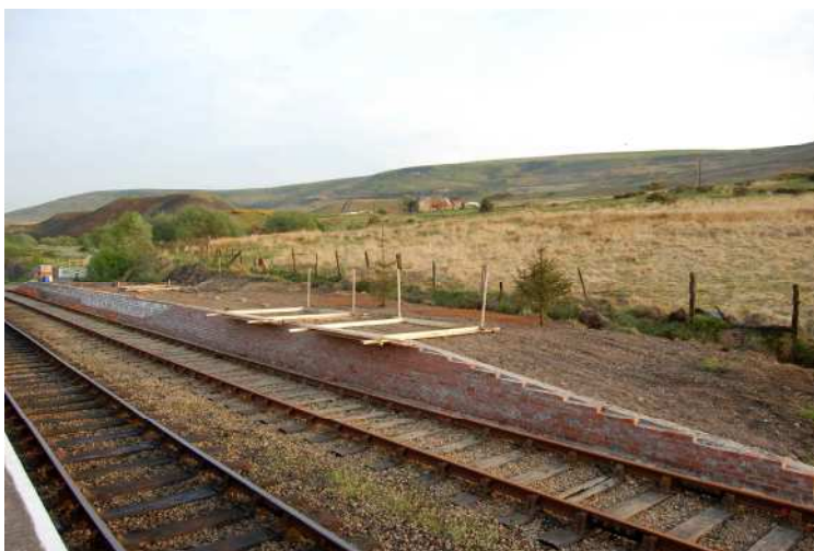
The north end of platform two showing the brick frontage, the completed backfill and the shuttering ready for the pouring of the concrete.
